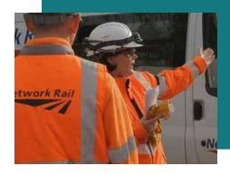
She tells the team which **line** is blocked and protected and which one is **open to traffic**. For both, it's important to know the **maximum speed** of the trains that run on the lines.
