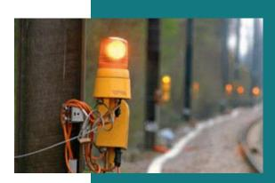
With an **Automatic Track Warning System** (ATWS), approaching trains are detected by equipment attached to the running rails.
