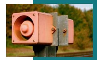
With a **Train Operated Warning System** (TOWS), approaching trains are detected by the signalling system.
