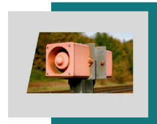
We also use four types of **equipment warning** systems. With Equipment Warning you will be warned when a train is approaching. The COSS or the Safe Work Leader will make sure enough prior warning is given for you to reach the position of safety. You must be in the position of safety at least 10 seconds before the train passes.
