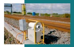
With a **Look Out Operated Warning System** (LOWS), the warning system is activated by the Look Out when a train is sighted. The warning is given by trackside flashing lights and sirens and/or a personal warning device.
