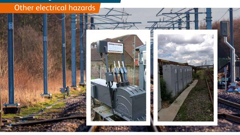
Electricity at the trackside is also present as the electrical supply for the signalling equipment. It is typically contained within a location case, supply terminal pillar, relay room or Functional Supply Point (FSP), but we can refer to them all as FSPs (as shown in the pictures).
