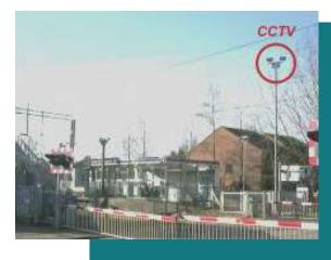
A **CCTV level crossing** is one that is controlled by a Signaller in a signal box. They close the road barriers whenever a train is approaching. Once it has passed the barriers open again. The Signaller uses CCTV to monitor what's happening at the crossing.
