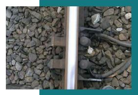
If counter heads become damaged, it can mean that a signal becomes stuck on red.
