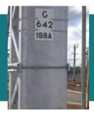
This is an overhead line equipment or **OLE structure**. Its number can be quoted to the Electrical Control Operator (ECO) in the event of an electrical emergency. Other structures such as bridges also have identification number plates.
