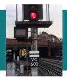
Most **signal posts** have a number which corresponds to the controlling signal box. You should give this number when telling someone (such as a Signaller) your location.
