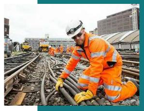
**Buried services** are cables or pipes laid under the ground carrying electricity, gas, water, and so on.
