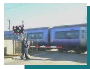
Automatic half barrier crossings operate automatically by detecting whether a train is approaching. As their name suggests, the barriers on both sides only extend across half of the road.
