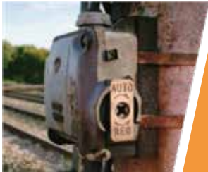
A signal post replacement switch
